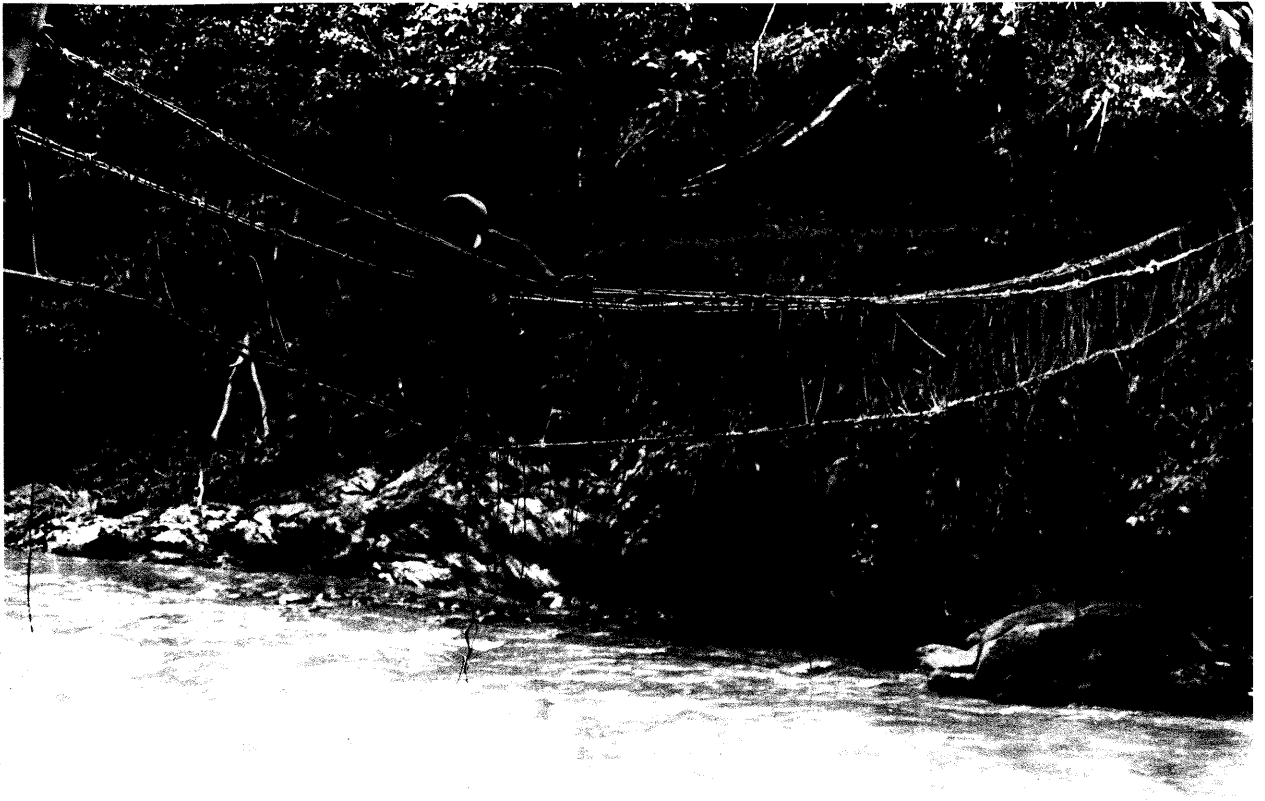
Photograph 2. Cane bridges such as these make travelling hazardous.
